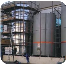
Insulation & Cladding of Tanks
